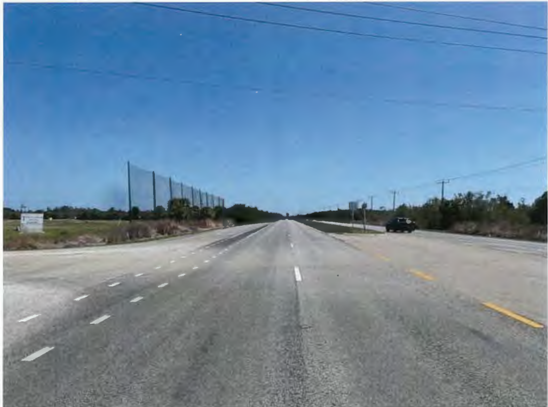
Looking south from the intersection along SR 951
