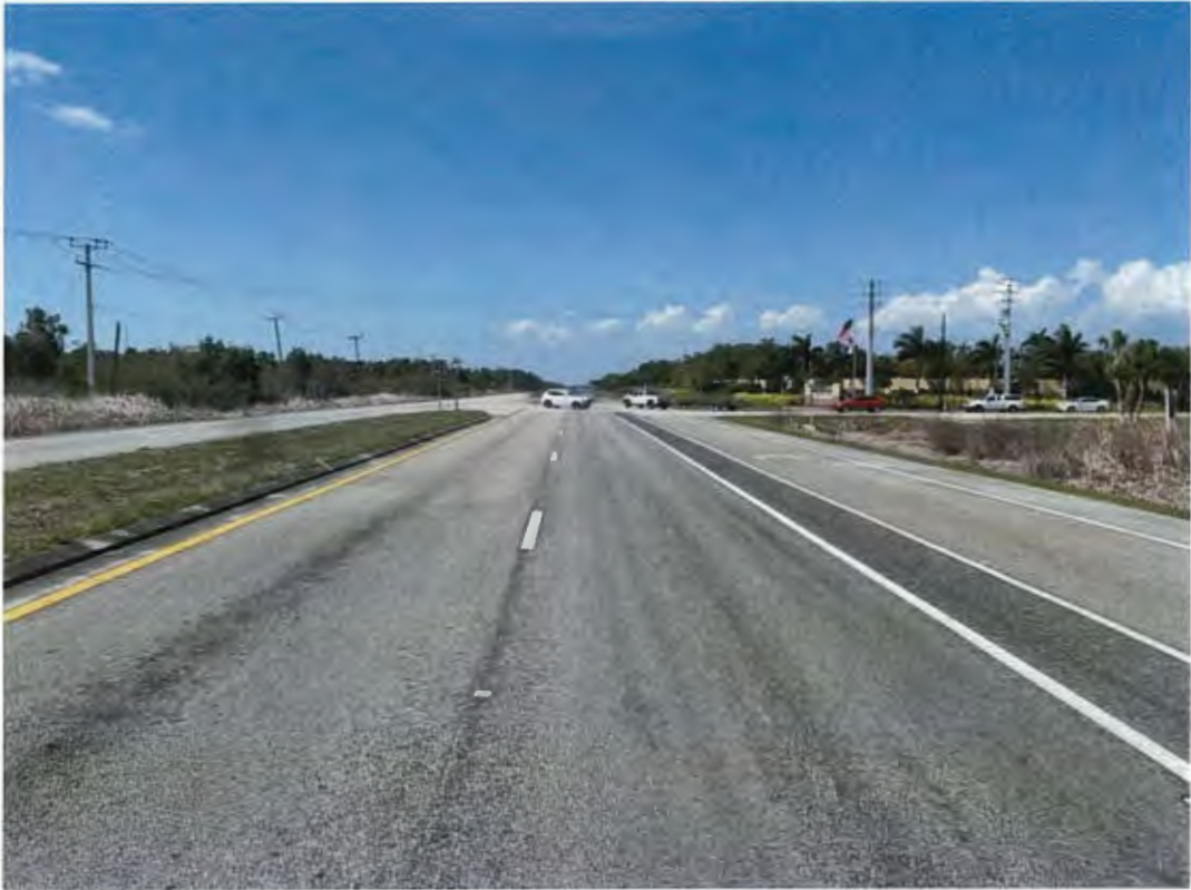
Looking north at the intersection along SR 951
