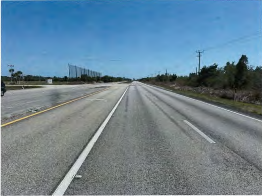
Looking south at the intersection along SR 951
