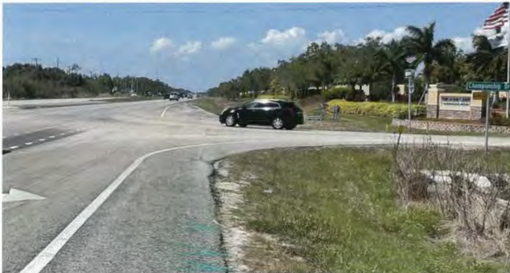
Looking north along SR 951 at a WB right turn from the SE quadrant
